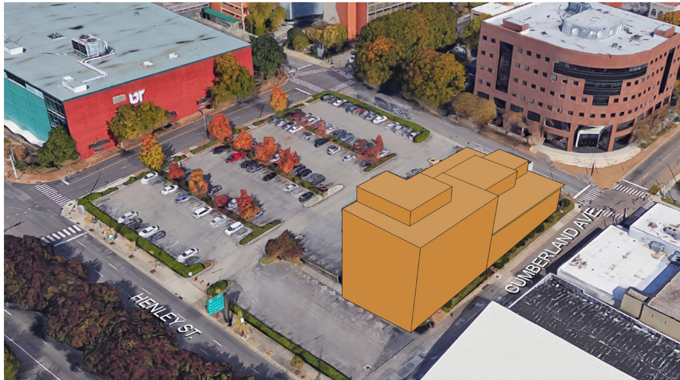
CURRENT DEVELOPMENT SITE W/ EXISTING STRUCTURES
