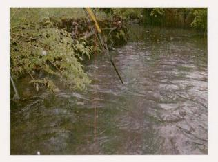
On April 4<sup>th</sup>, 2008 staff members Jake Hudson and Scott Wilson removed this blockage on Williams Creek. The weir was made up of one large log that stretched from one shoreline to the other, many small limbs, one large sign and one bag of trash. The trash and woody debris was pinned against the guy-wire and blocked a majority of the creek. The wood was removed and the trash and sign were collected and removed from site.
