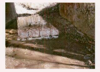
This weir was removed on December 4, 2007 by staff members Jake Hudson and Scott Wilson. Two trees and several large branches were blocking about 40% of the creek and redirecting the flow to the east bank. The trees were removed using a chainsaw. The branches were collected and removed, opening up the flow of the creek.
