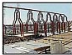
Construction site of the new Knoxville Convention Center (taken 2-29-01)
