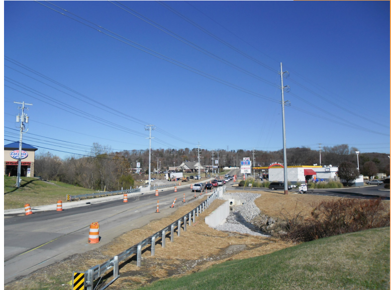
Millertown Pike (During Construction - Looking Northeast)
