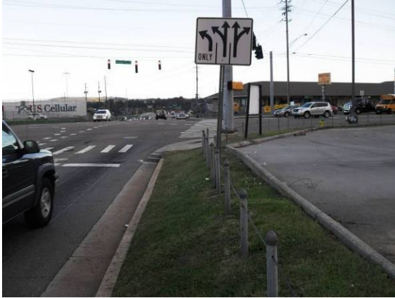
Gallaher View at Kingston Pike Before Construction
