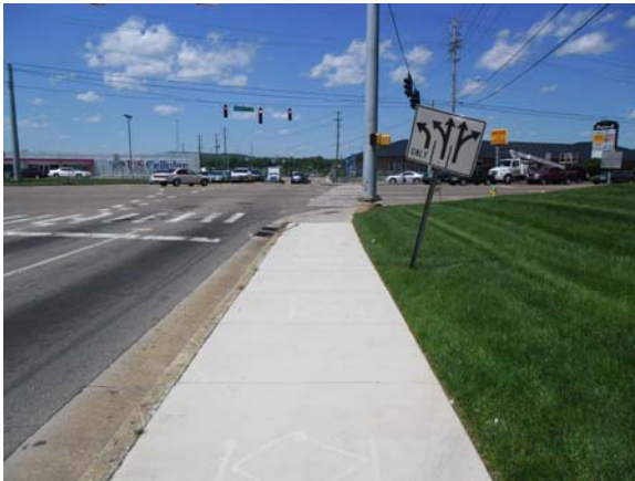
Gallaher View at Kingston Pike After Construction
