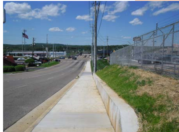
Gallaher View Road Looking North After Construction
