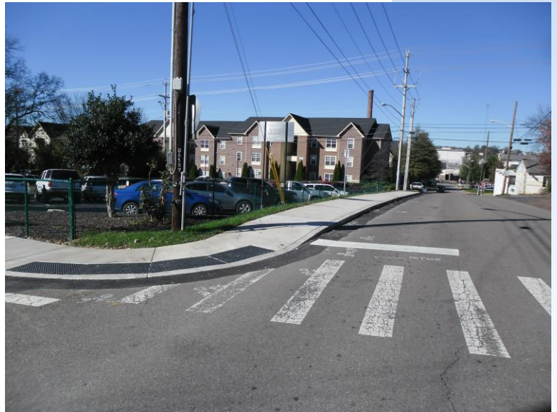
S Twenty Third Street from Highland Avenue Looking South - After Construction
