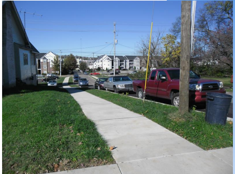
S Twenty First Street from Highland Avenue Looking South - After Construction
