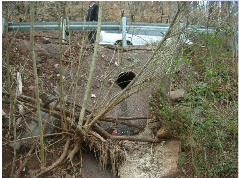
Existing Drainage Pipe Under Cherokee Trail
