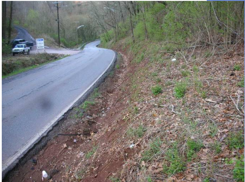
Cherokee Trail (Before Construction – Looking West)
